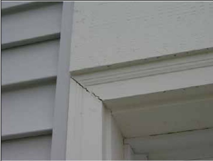
Caulk wood trim
